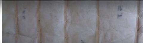
Compression or incomplete fill amounting to 2% or less, if the empty spaces are less than 30% of the intended fill thickness, are acceptable for “Grade I”.
