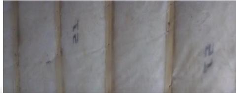
2. “Grade II” shall be used to describe an installation with moderate to frequent installation defects: gaps around wiring, electrical outlets, plumbing and other intrusions; rounded edges or “shoulders”; or incomplete fill amounting to less than 10% of the area with 70% or more of the intended thickness (i.e., 30% compressed); or gaps and spaces
